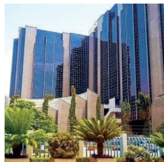
Central Bank of Nigeria Abuja, 2001
